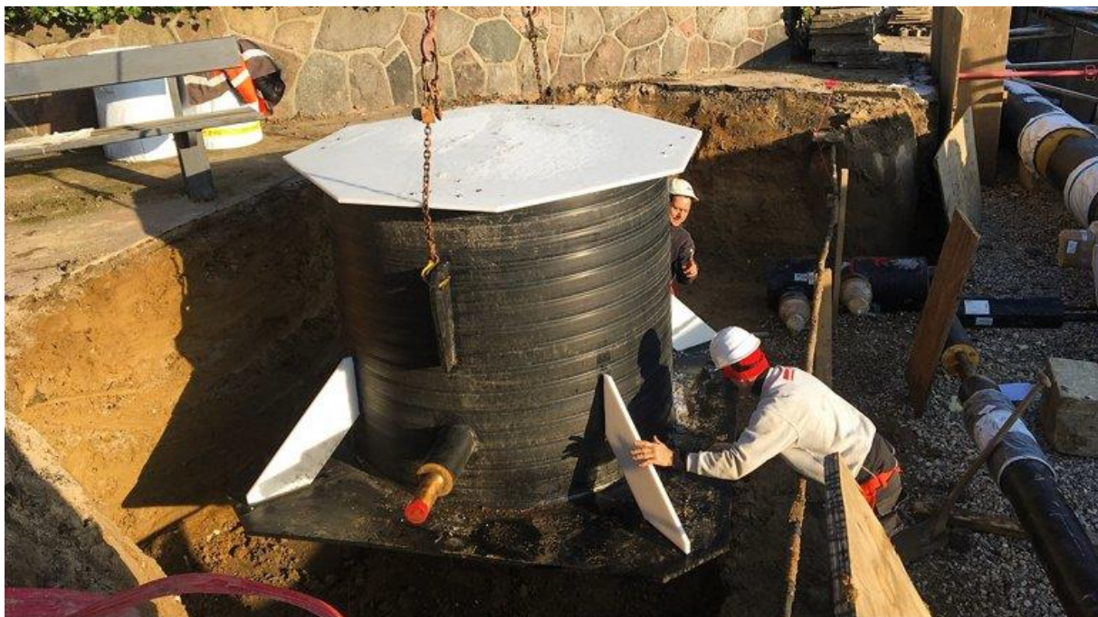
Figure 56: Installation of shunt connection in Gentofte (source: Grundfos) 29 .
