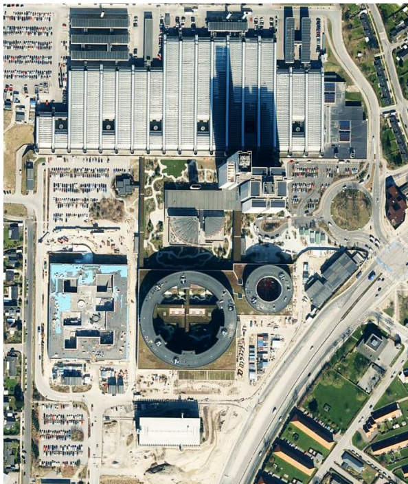
Figure 57: Herlev New Hospital (Denmark)
