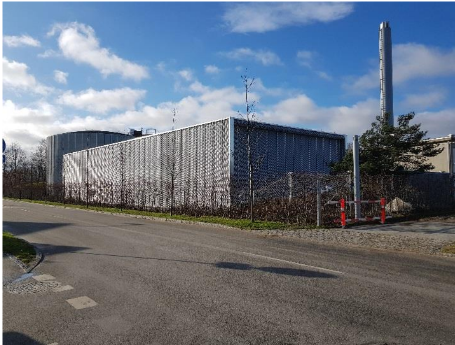
Figure 60: Heating plant in Taarnby District heating and Cooling system.
