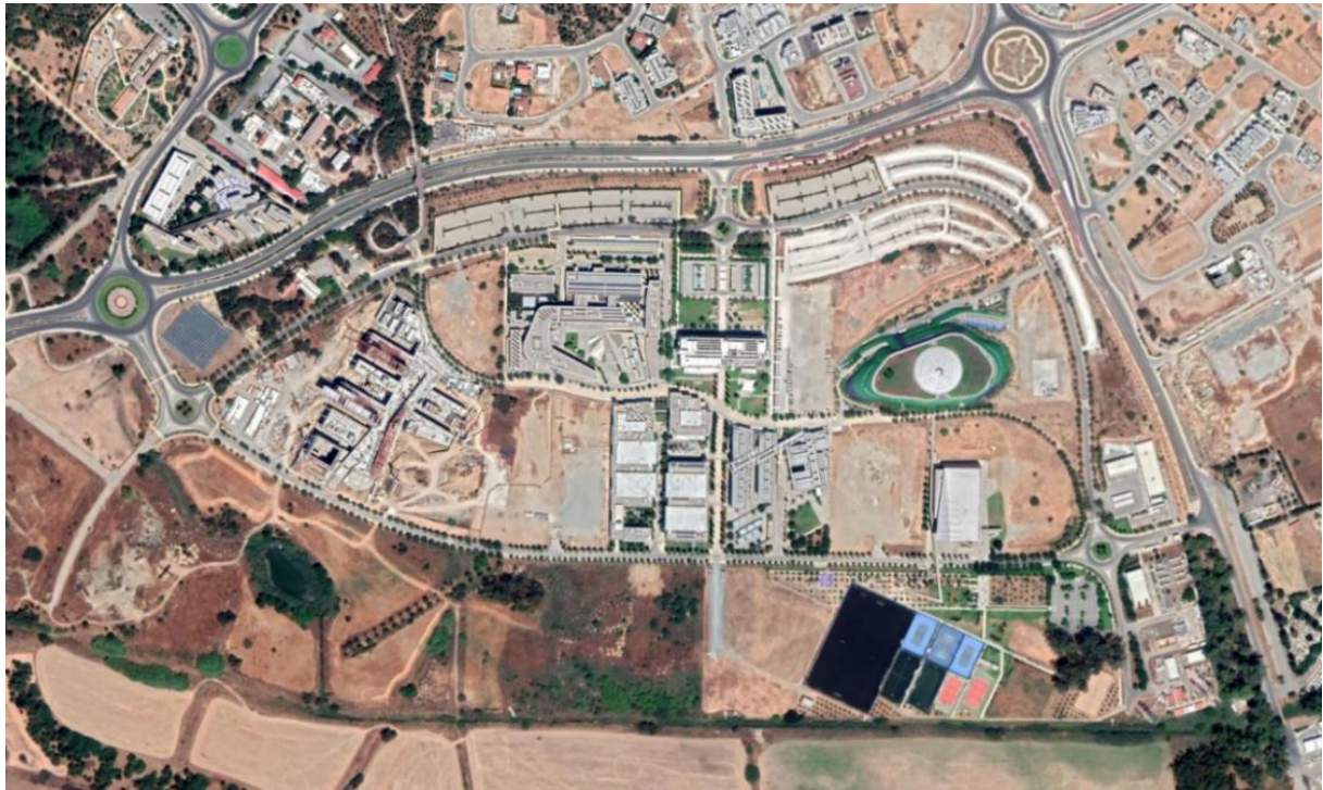
Figure 4-26. University of Cyprus – Aerial campus photograph.
