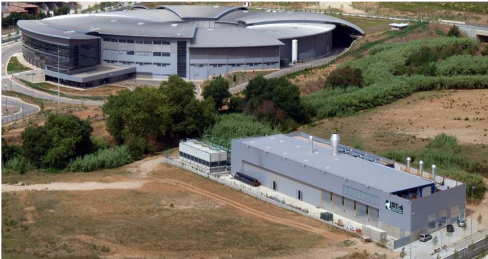
Figure 4-1: Parc de l'Alba main generation plant (foreground) and Synchrotron (background)
