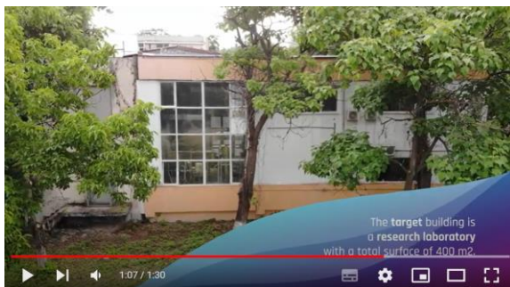
Figure 10 – Screenshots from first demo site video at Bucharest on YouTube showing the ground works on UPB campus.
